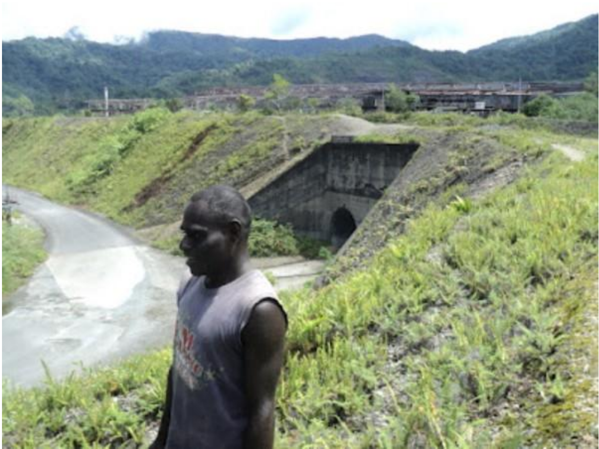
Public vehicle pit area access tunnels
