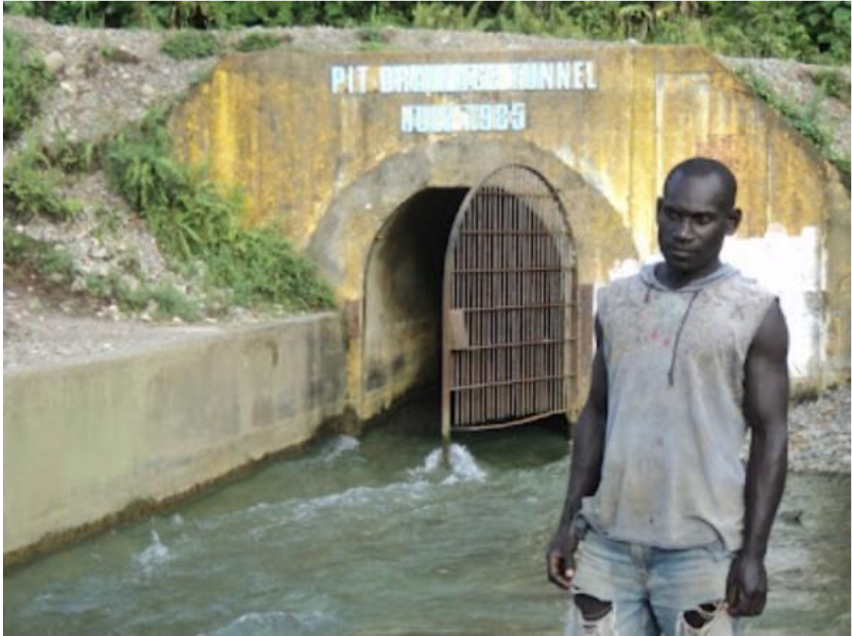
Pit Drainage tunnel entrance
